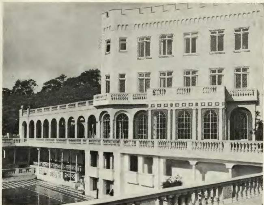
The Residence. Colonnade and Courtyard
