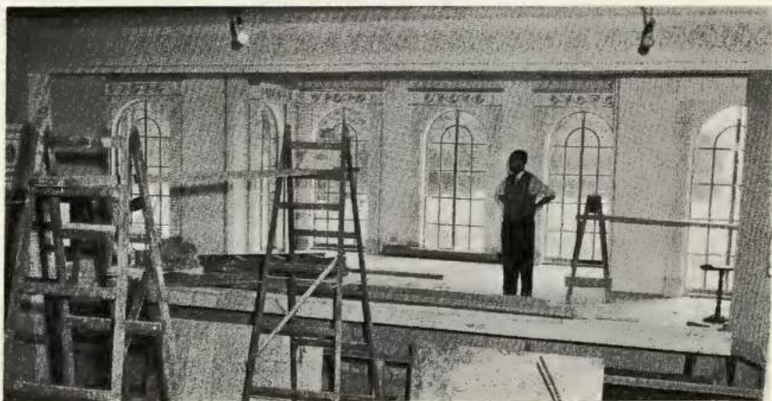
Work during construction of the Private Theatre
